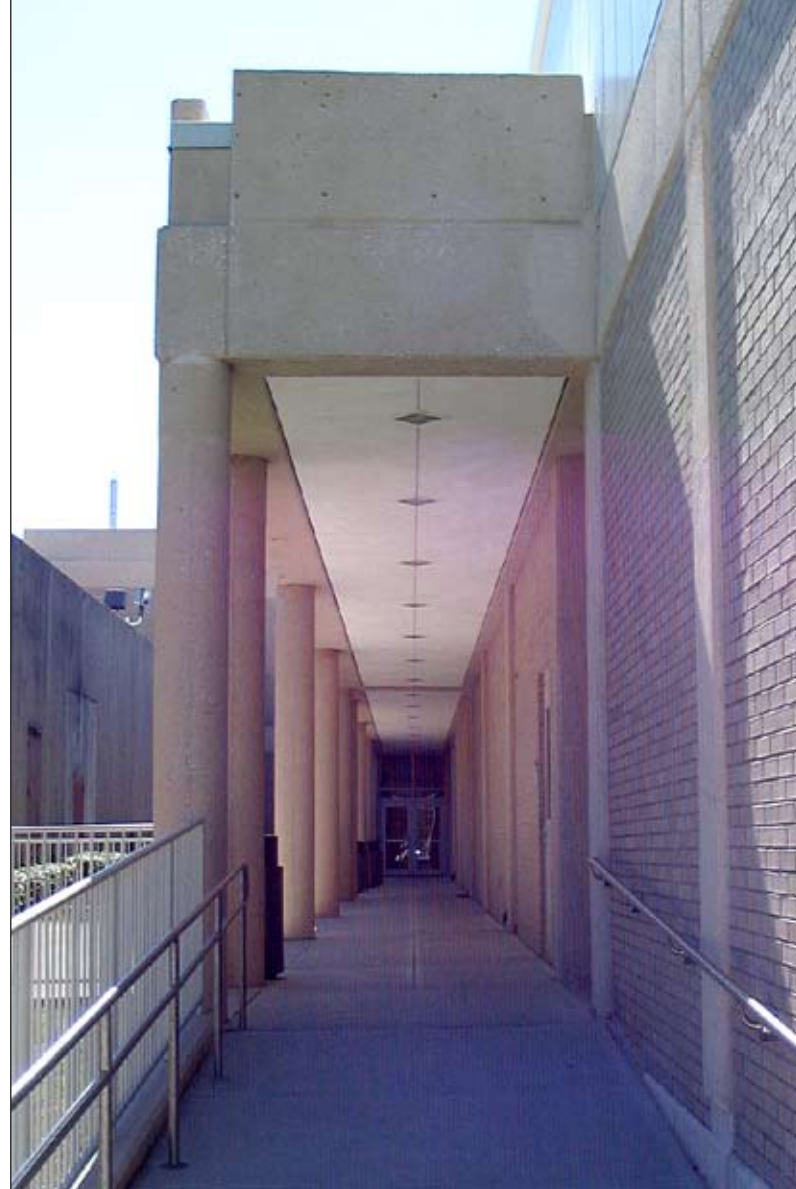
Arcade at the Engineering Building
