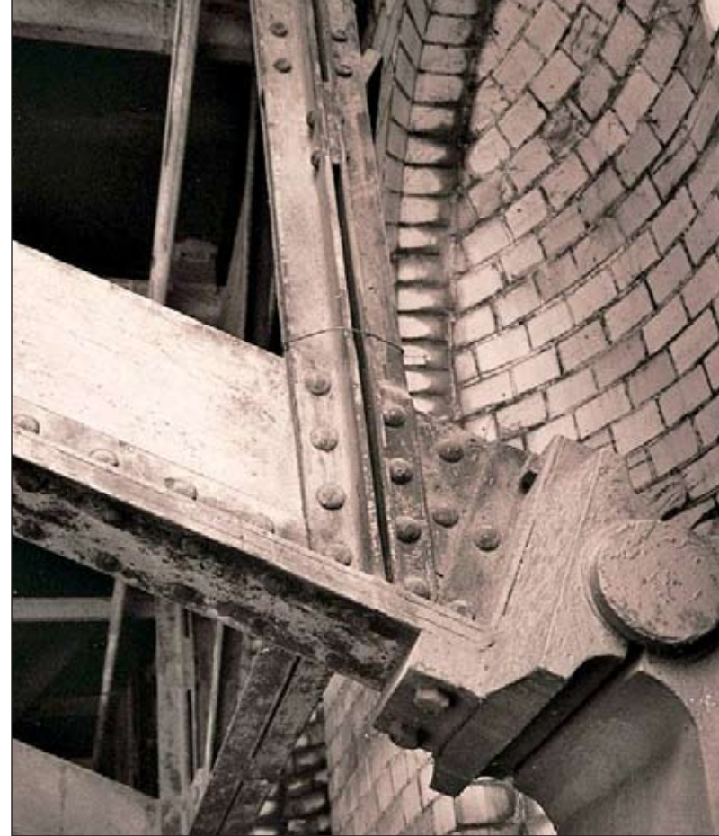
Masonry and steel
