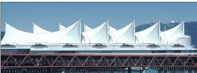
Sail-like building construction
